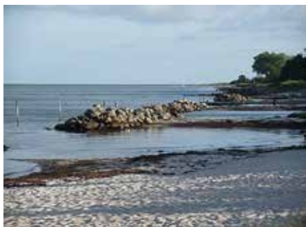
Breakwaters at southwestern Baltic Sea coast
