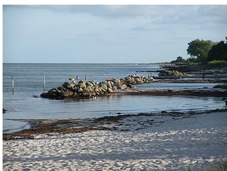
Breakwaters at southwestern Baltic Sea coast
